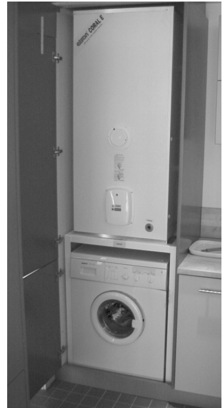
Typical Coral E WMF installation
